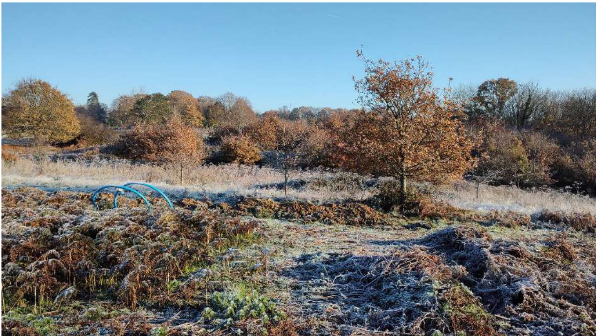
Plate 10: Pod erection site with service trench and spoil heap (dir. E)
