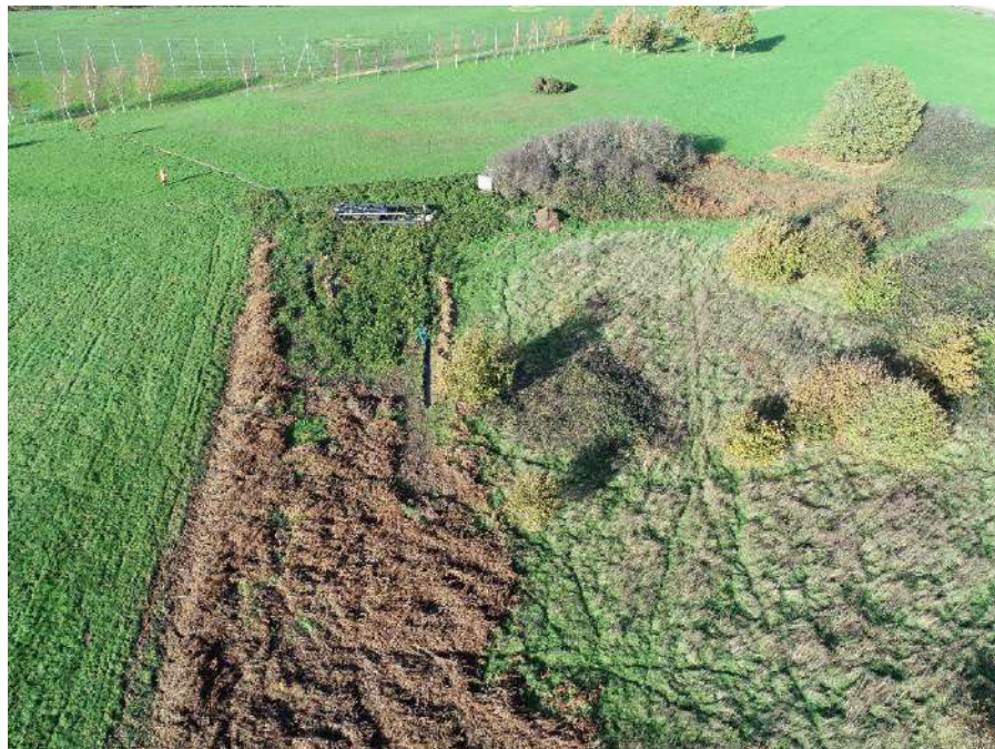
Plate 14: aerial view of the pod installation site (dir. N)
